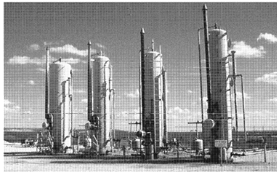
Figure 4. Two of the heater/treaters can be owned by the operators and the third reserved for treating oil in the tank battery. The fourth is used for well testing.
