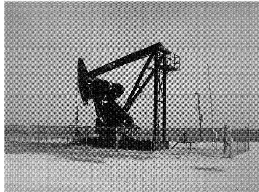
Figure 5. A security fence has been installed around this pumping unit because the well is near a busy highway.
