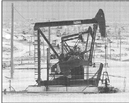
Figure 8. The Mark II Uinitorque Pumping Unit.
