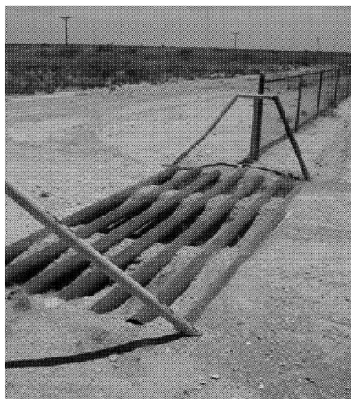
Figure 3. A poorly maintained cattle guard.
