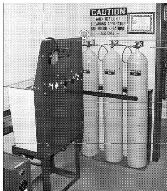
Figure 6. Industrial-sized bottles awaiting to be refilled. The water tank to the left is used to cool smaller bottles when they are being filled.
