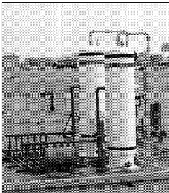
Figure 3. Injecting chemicals at the tank battery.
