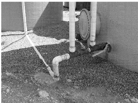
Figure 5. The basic water disposal system involves draining the water from the gun barrel and moving it through a line to the water disposal tank.
