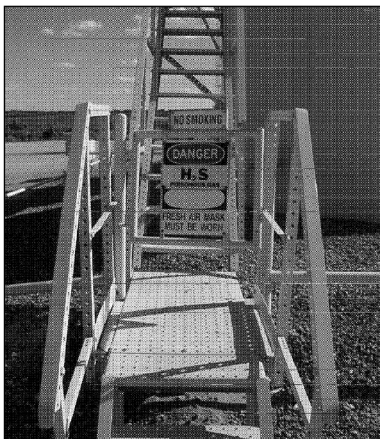
Figure 2. A warning gate that indicates the presence of H 2 S and the requirement for breathing apparatus.
